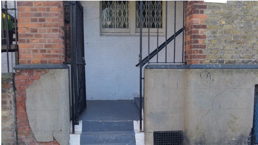
Fig 7.1 Access to hall via fire exit with 4 steps.
